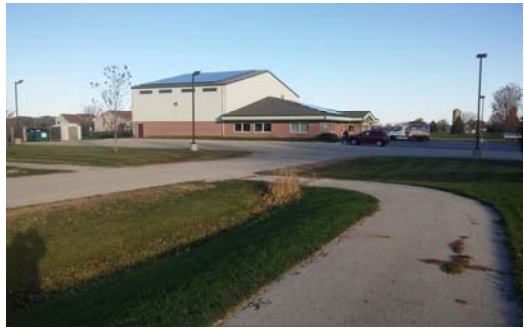
COUNTY H RECREATION CENTER, 41 KILOWATTS
