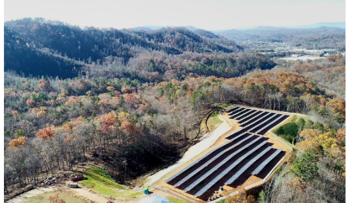
A 705-kW solar array installed near the EBCI-owned casino in Murphy, North Carolina. Photo by Joey Owle, Eastern Band of Cherokee Indians
